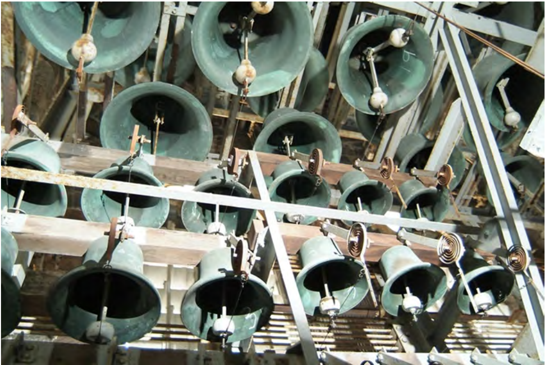
Fig. 38. The carillon of 48 bells cast by G&J in 1951 and 1954.
