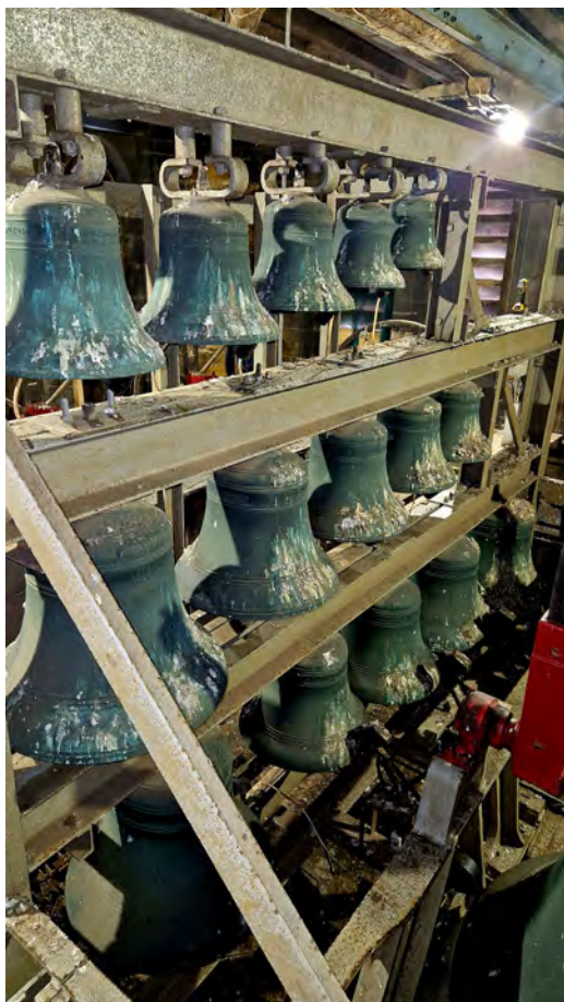
Fig. 14. The new casting of eleven bells and the four 1932 clock bells were hung together in a vertical steel frame inside the outer bellframe housing the ringing bells in 1951. They are now sounded by electro-magnet hammers mounted inside each bell. This is the installation as it existed in 2024.
