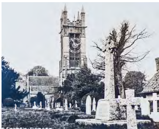
Fig. 21. Early twentieth-century photograph of St Peter and St Paul's Church, Cattistock, Dorset by an unknown photographer. The very large skeleton dial was installed by Gillett and Bland; it was much criticised at the time because of its large size.
